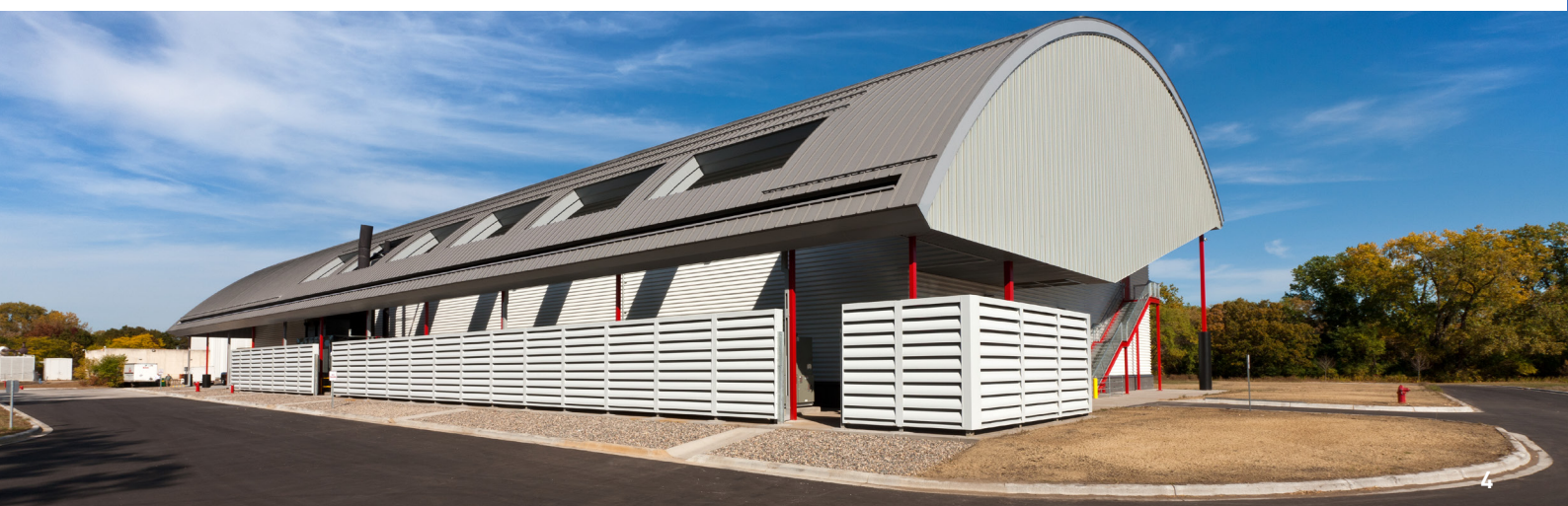
Ventilation system for air intake and/or exhaust equipped with acoustic louvers
